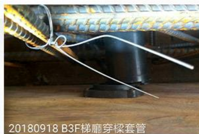
B3F梯廳穿樑套管脫落
